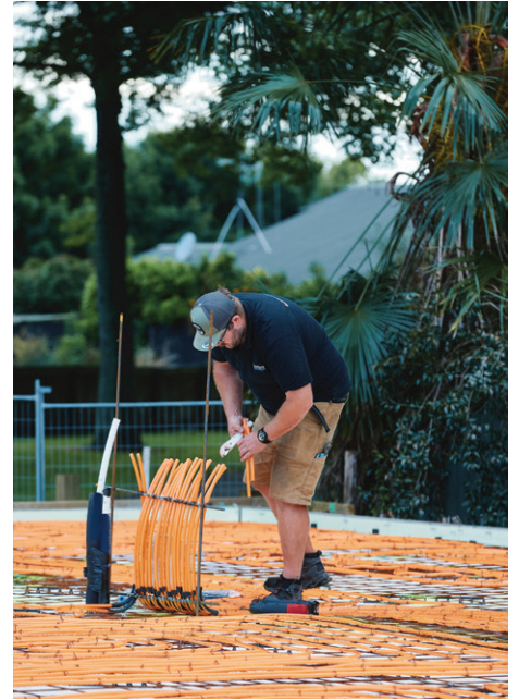
— Underfloor installation
