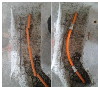
Large section of pipe cut and repaired
