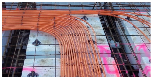
Underfloor install showing "hot track" of grouped pipe
