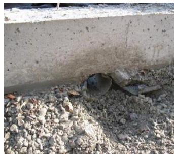
Pipe penetration through foundation wall
