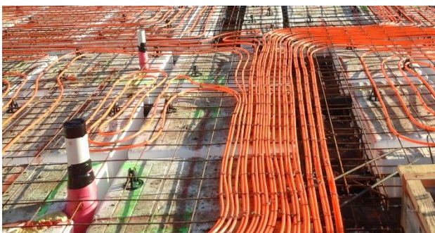
Underfloor install showing "hot track" of grouped pipe
