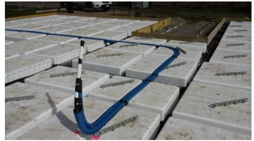
Feeds through rib-raft slab
