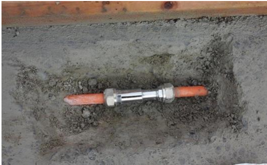
Pipe repair using telescopic connector (option 1 above)
