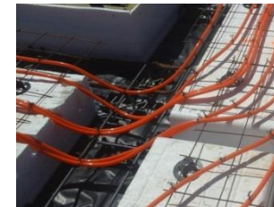
Pipe dipped below section of mesh
