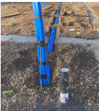
Feed pipes rising vertically, trenched through hard fill
