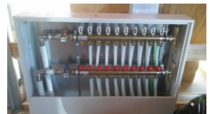
Optimal feed pipe placement in cabinet
