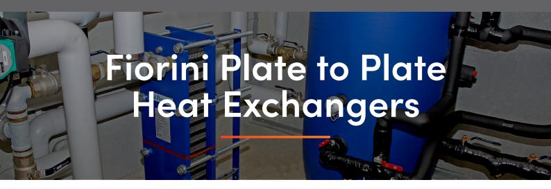
At Central Heating New Zealand, we provide versatile and efficient heating solutions, with Fiorini plate to plate heat exchangers exemplifying this dedication. Engineered for high thermal efficiency, these units facilitate optimal heat transfer for residential and commercial applications, including process heating. Their design uses a series of plates to create a large surface area for effective energy exchange between two fluids, minimizing energy loss and reducing operational costs.
