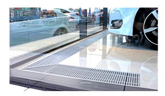
Trench convectors are a great solution for spaces with large amounts of glazing such as living spaces and retail showrooms, with the heat being delivered directly
