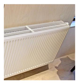
One aspect that needs to be considered when using radiators in sensitive commercial spaces such as hospitals, childcare and elderly care centres, is the radiator surface temperature. As per building clause G5.2.2, appliances must be installed in a way that reduces the likelihood of injury. In these types of projects the inhabitants could be immobile and if resting up against a radiator with 80°C water flowing through it, scalding could be a real concern after a period of time.
