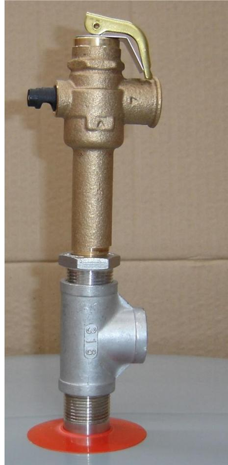
TPR fitted with Tee and reducer. 240mm is needed above top surface of the cylinder to allow enough room to test the TPR.
