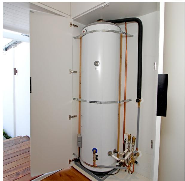
2. Electrical immersion element permanently set to at least 60°C with ripple control power supply. Use of domestic hot water will cause tank temperatures to fluctuate, lower tank temperatures will fall as low as 10–20°C in normal usage with reheat times of around 1–2 hours before the entire tank contents is heated back to 60°C. Reheat times can be longer if usage is during peak tariff periods and element is off.
