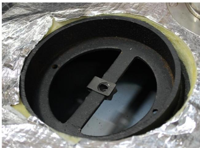
Use the white fibre gasket in the flue kit with the standard efficiency boiler.
