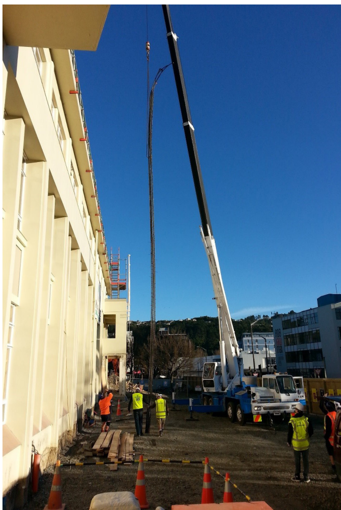
The test pile being lowered into position
