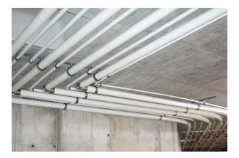
Pipe work must have a lifetime in excess of 50 years, have a maximum operating temperature of 95°C @ 7 Bar and a maximum operating pressure of 10 Bar. The pipe work must be installed in accordance with the manufacturer's guidelines. Pipe joints to be avoided within the slab at all times.
