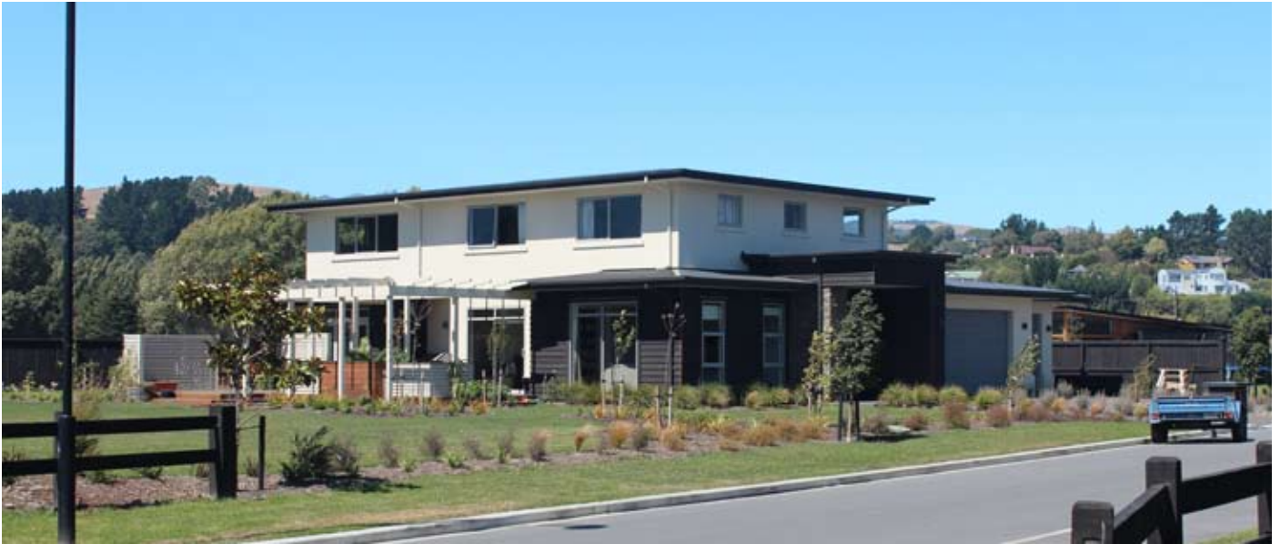
This newly built home features radiators and an air-to-water heat pump.
